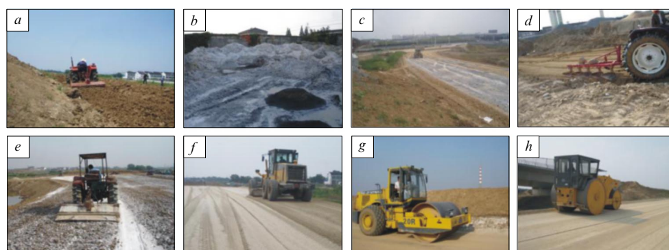
Figure 32. Construction of CCR-amended Embankment. Placing and spreading filled soil (a); tedding and air-drying CCR (b); paving CCR by scrapers (c); mixing CCR and filled soils by a plow 1LF-335 (d); enhanced mixing CCR and filled soil by a dozer (e); grading CCR-amended soil (f); compacting CCR-amended soils by a vibratory roller SR20MP-2 (g); enhanced compacting CCR-amended soils by a steel-wheel roller YC6108G (h). Reproduced with permission of the authors of Ref. 265.
